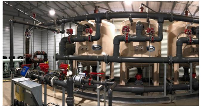
*The new state-of-the-art Layne AIM treatment plant removes arsenic, iron, and manganese from the water at the rate of 1,200 gallons per minute.*
