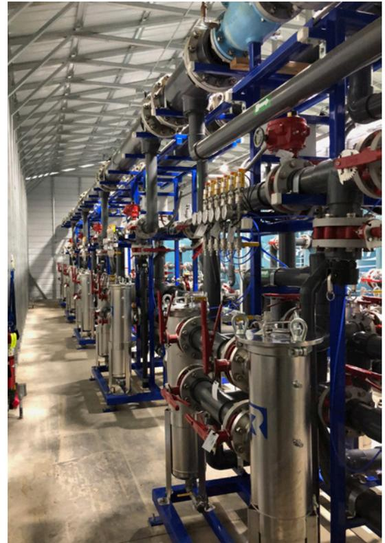
*The new state-of-the-art WRT treatment plant removes uranium from the water at the rate of 1,000 gallons per minute.*
